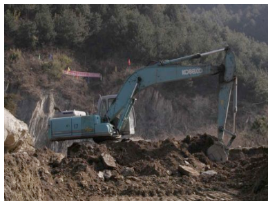
Construction of the Tudiling Tunnel begins ©WWF China
