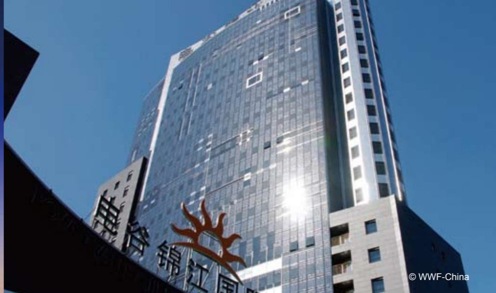
● Baoding's Power Valley Jinjiang International Hotel is partially powered by self-generated solar electricity, which comes from nearly 4500sqm of solar panels that have been design. 保定电谷锦江酒店是中国首座太阳能五星级酒店，安装的4500平方米的太阳能面板所产生的电能，可以部分满足酒店的用电需求。
